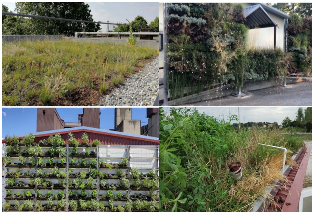
Figure 21. Top left: overview of the Green Roof realized on the WOW building in Turin (image © City of Turin); top right: the Green Wall realized on the homeless dormitory in Turin (image © City of Turin); bottom: the seedling factory with the green wall (left) and the green roof (right) (image © M. Ristorini and A. Campiotti).
